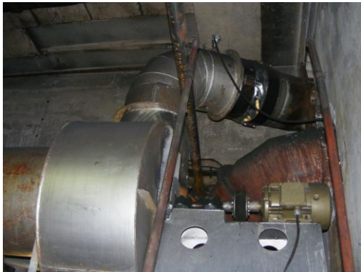
Fig 4. An example of flexible connection
