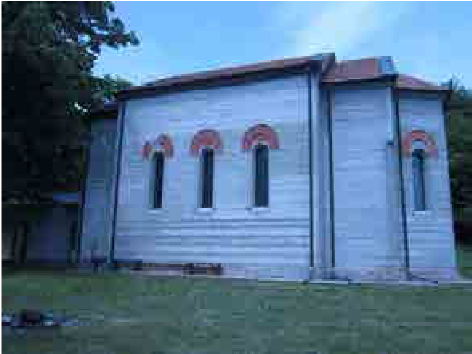
Fig. 6. Exterior of the monastery (by M. Milojević)
