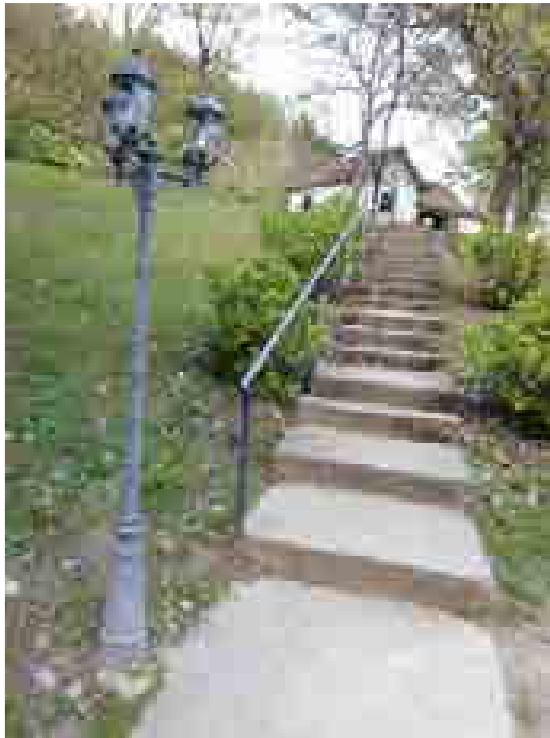
Fig. 4. The stairway between the chapel and the resting point for the guests
