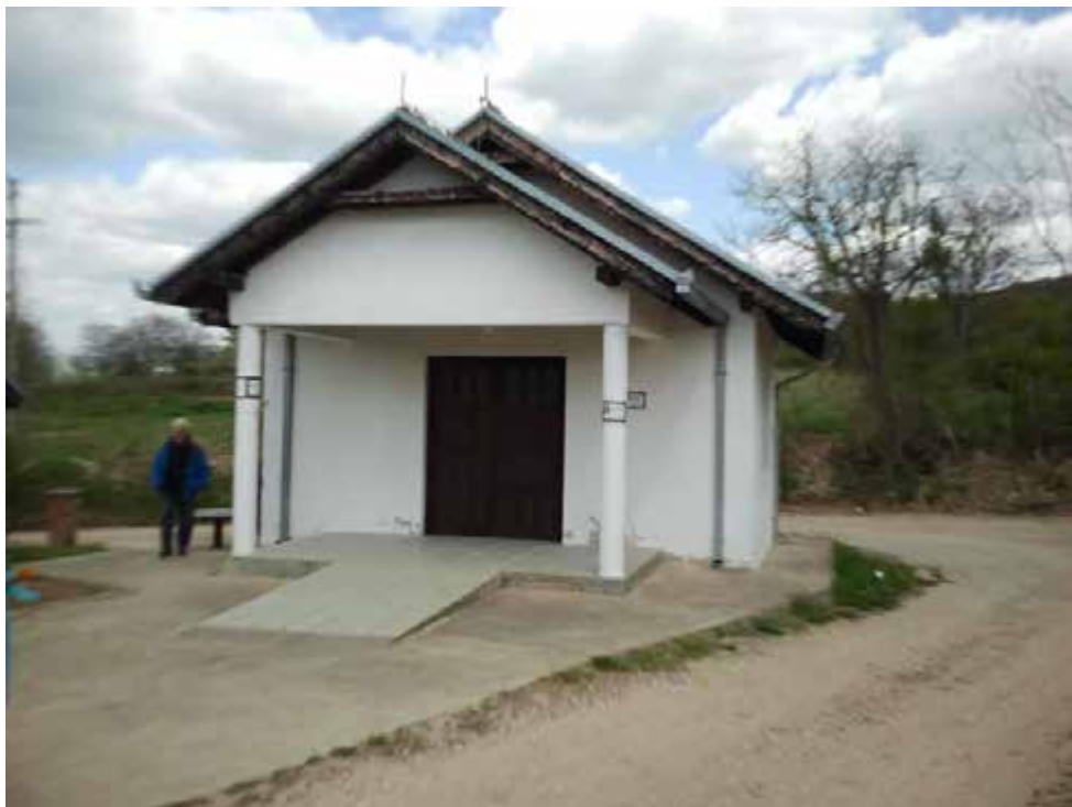
Fig. 3. Chapel, view from the courtyard of the cemetery
