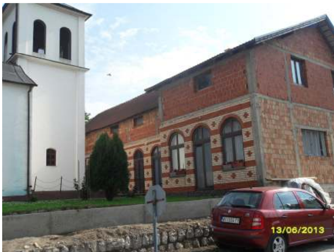
Ph. 9. The works on the parish home
