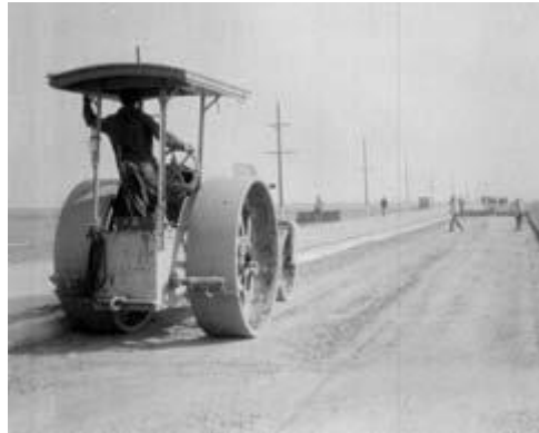
Figure 2.a 1930s: A form of RCC paving is performed in Sweden
