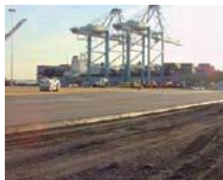
Figure 2.c. Late 1980s–early 1990s: RCC pavements are constructed for automotive, port, and intermodal facilities in the U.S.
