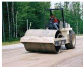
Figure 2.b. 1970s: RCC pavements become common for log-sorting yards in Canada
