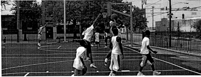
Figure 4. Herron Recreation Centre, South Philadelphia. Basketball court with porous paving and playground after project completion. Directly below the basketball court's porous asphalt surface is a storage tank composed of separate stone cells which capture runoff. Each cell is graded so that captured runoff flows towards the rain garden. (Source: http://www.temple.edu/ambler/csc/t-vssi/bmpsurvey/herron_playgrd.htm )
