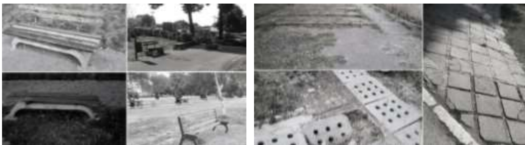
Figure 6. a) outdated and ruined mobiliard, b) destroyed paving
