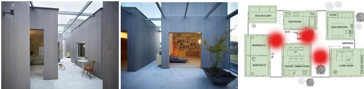
Figure 7 – House in Buzen, Suppose Design Office, Buzen, Fukuoka, Japan , 2009: photos (left), sketch showing integral volumes of the composition (green) and central gathering space (red) (right)*
