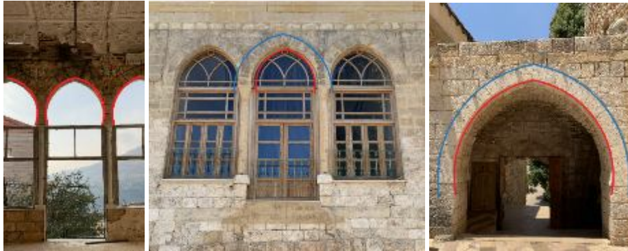
N) Example of pointed arch in: 1) three-arch houses (19 th c.) a) Bazoun, b) Baalbek, 2), c) Monastery of Saint Anthony kozhaia (19 th C.)
