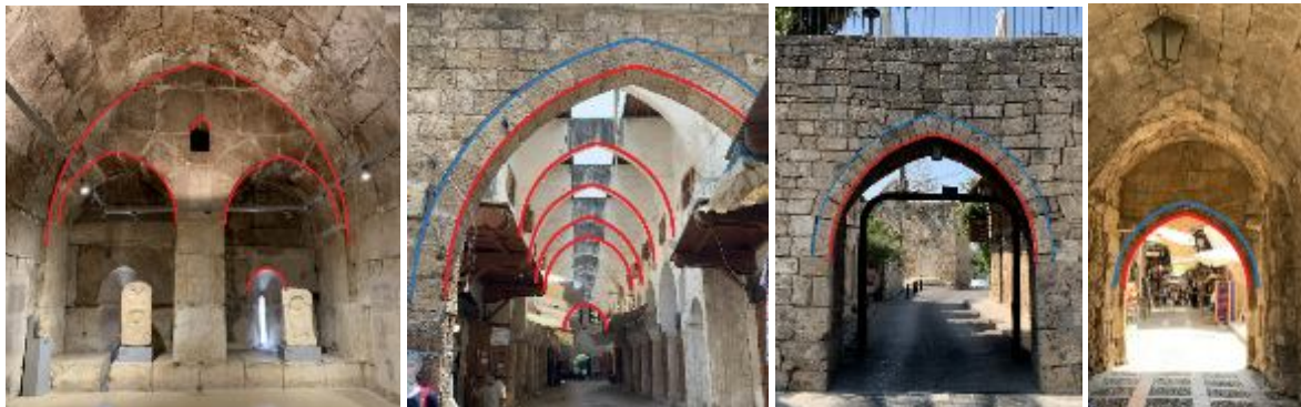
O) Example of pointed arch in: 1) Mamluck Architecture (12 to 16 th c.) a) Fortress in Baalbek, b) Market in Tripoli, 2), Crusaders Architecture (11 to 13 th c.) c) Door in the city wall of Byblos, d) Market in Byblos
