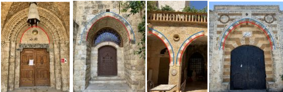
P) Example of pointed arch in: 1), a) Mamluck Mosque in Tripoli (early 14 th c.), 2), b) Palace of Fakhr Eddin II in Deir Al Qamar (17 th c.), d) Palace of Bachir II in Beit Eddin (18 th c.).
