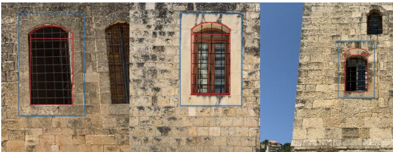
G) Windows respecting design E-a: a) 18 th c. in Beit Eddin palace, b) 19 th c. & c) 17 th c in Deir al Qamar
