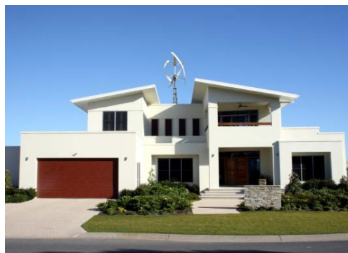
Figure 2. Retro-fitting wind turbines onto existing buildings, http://www.pljgroup.com
