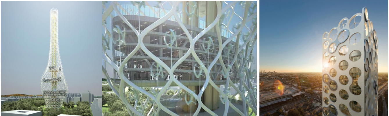
Figure 8. Taiwan Tower, http://www.designboom.com
